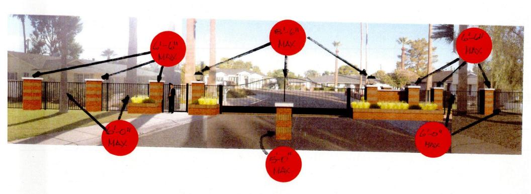
Note: Brick Columns Wave CHANGED TO Split FACE BLOCK WITH A BRICK RACING Stripe.
