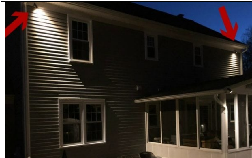
Figure 2 -- Lights can be placed under eaves and shine down to illuminate walls and adjacent areas
